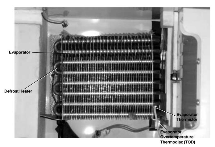
Figure 2 - Evaporator (Top of Freezer)
