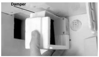
5. Carefully pull the damper out of the mullion and remove.
