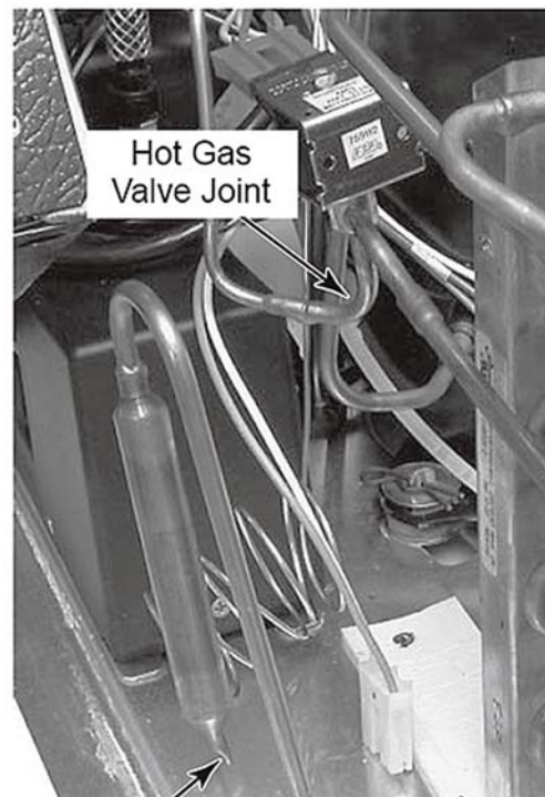
Drier Filter Capillary Tube
